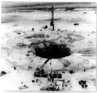
Compaction grouting was used to seal this 160-foot diameter sinkhole that extended down to the Floridan aquifer.
