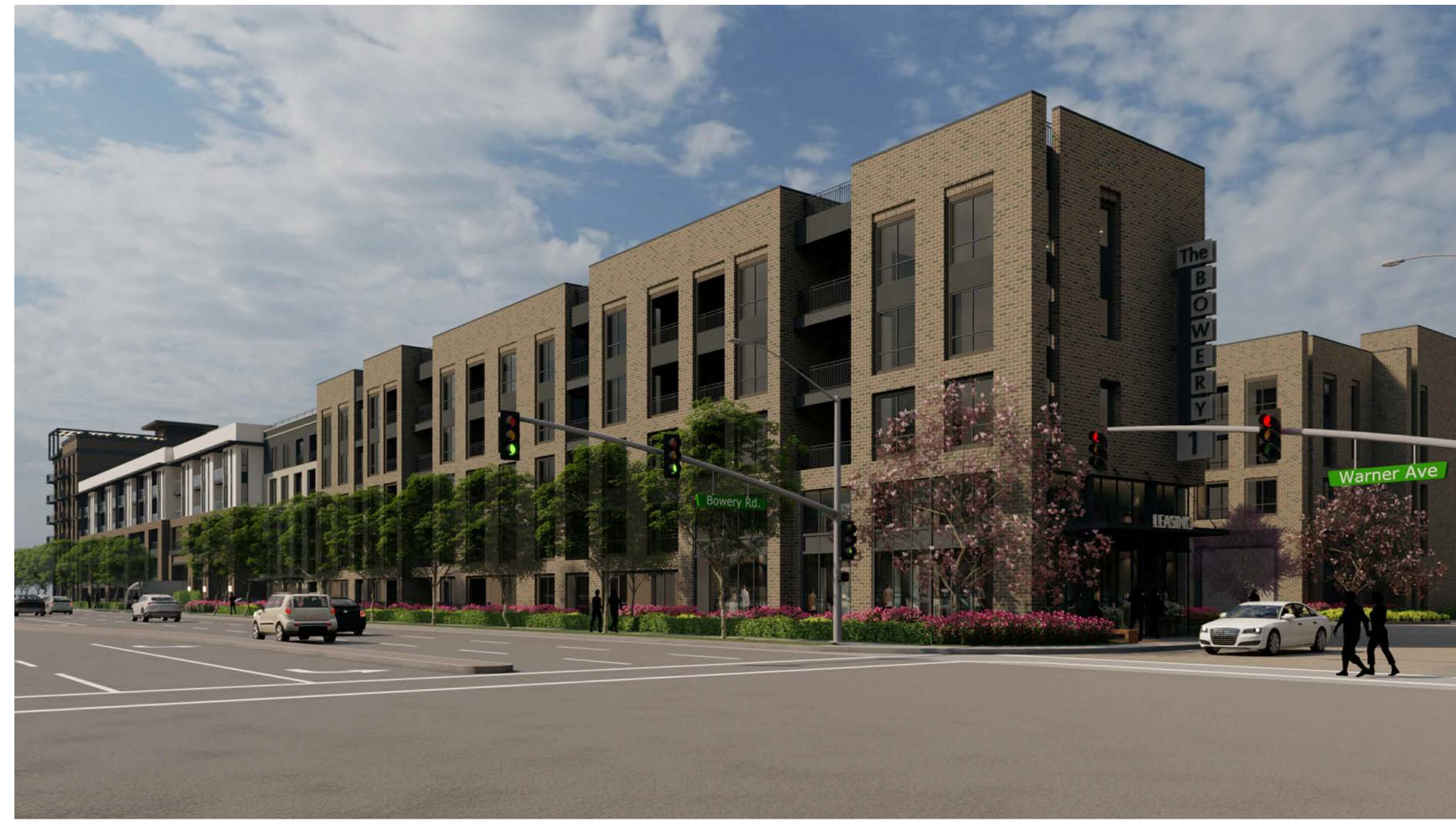
BLDG.'A' LOOKING EAST AT LEASING OFFICE 2
