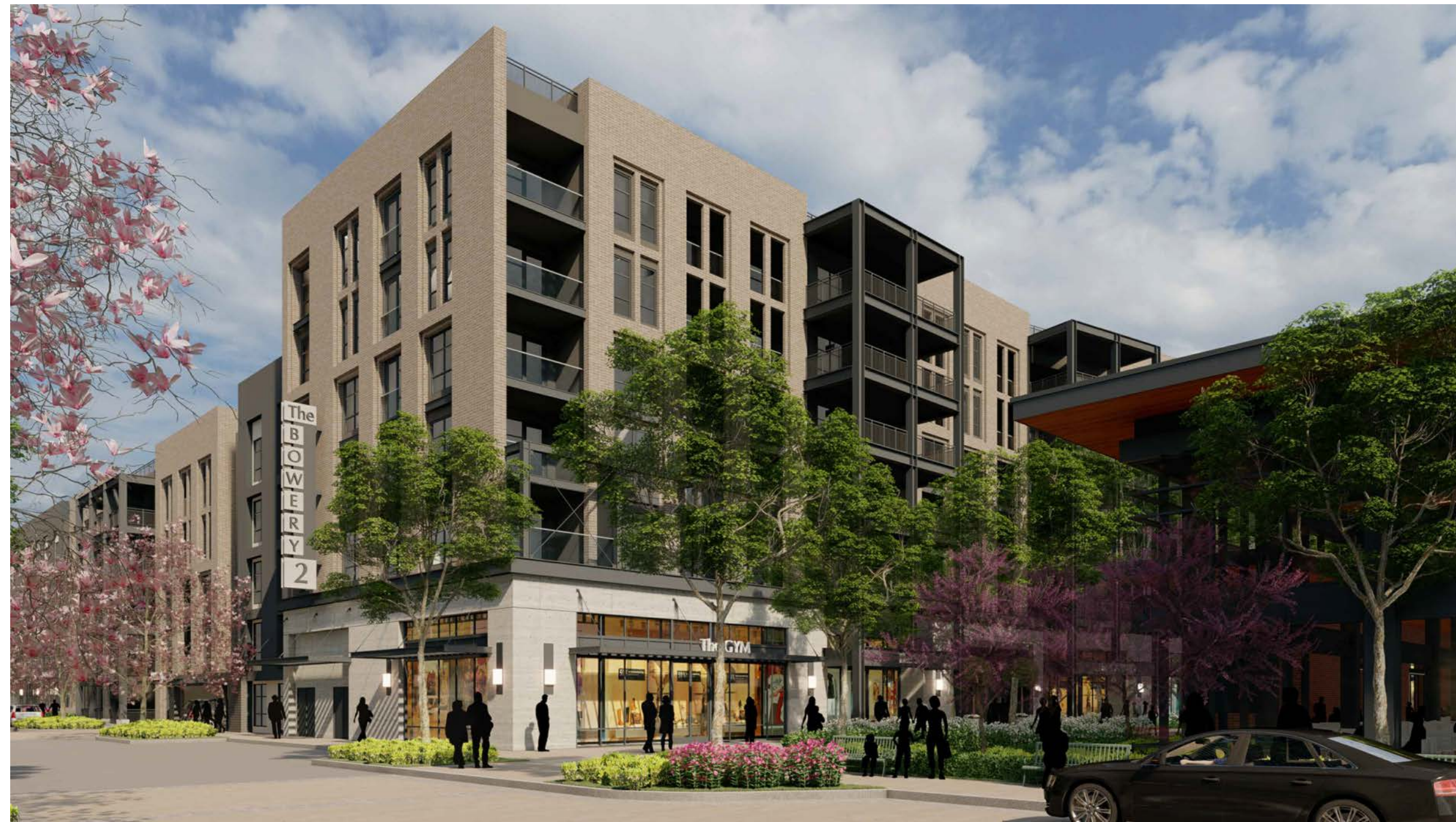
BLDG.'B' LOOKING WEST 3
