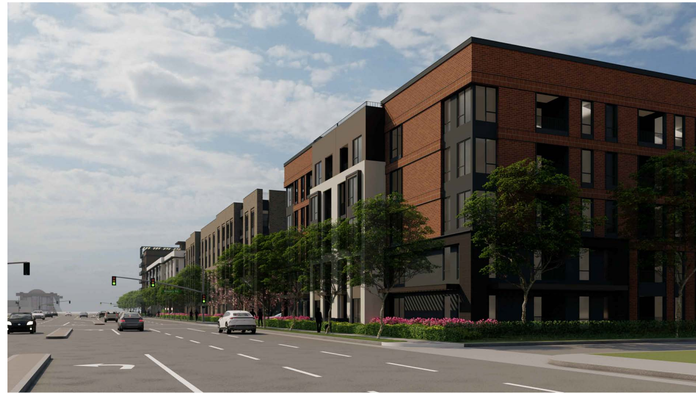
VIEW AT NORTHWEST CORNER LOOKING EAST 2
