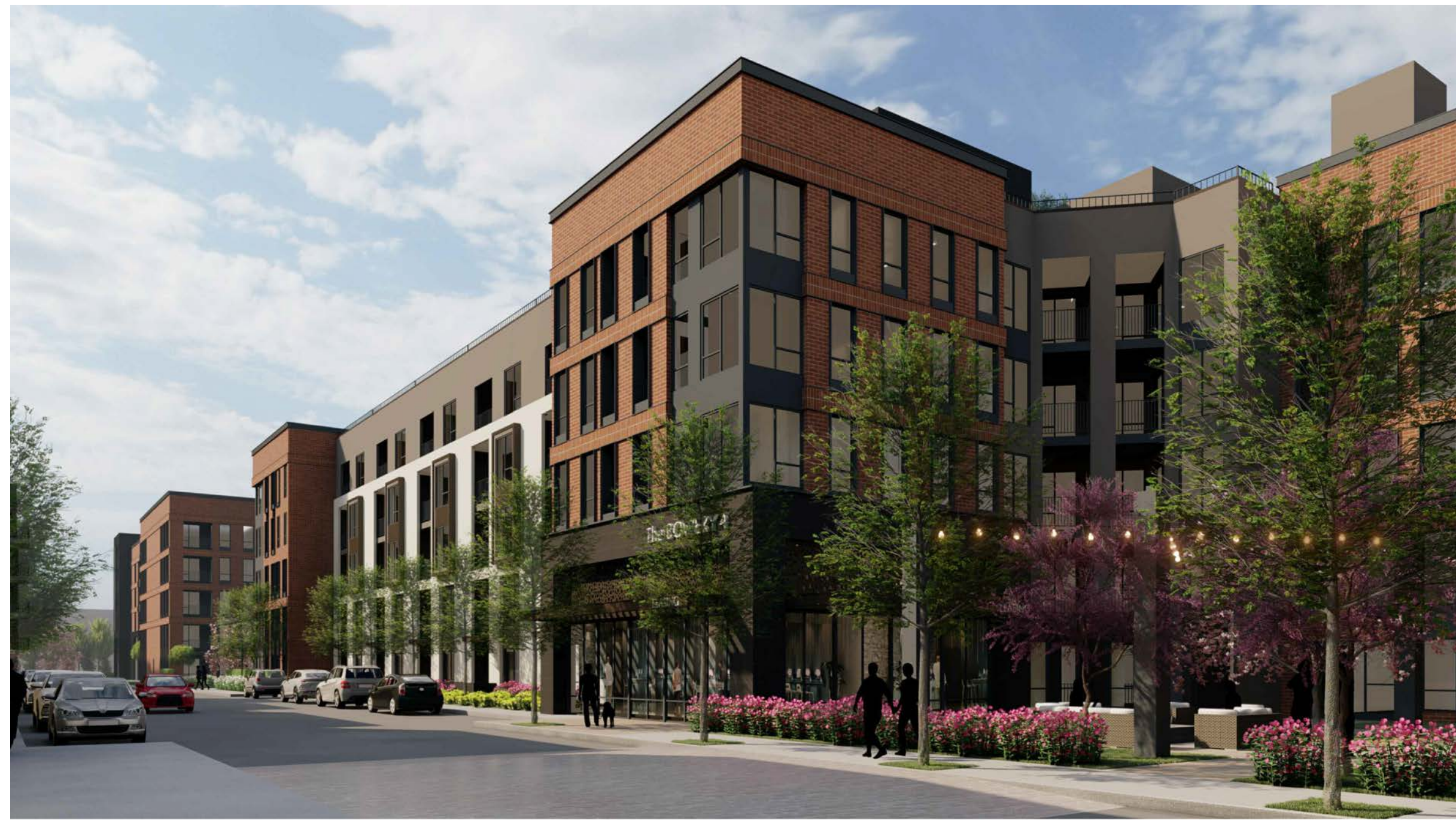
BLDG.'D' LOOKING WEST AT LEASING CENTER 4
