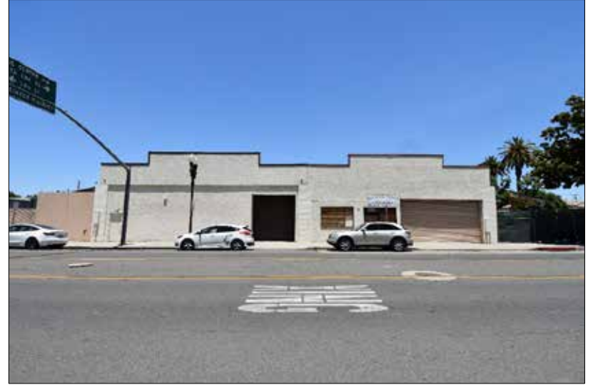
Southern View of Site B from 4th Street
