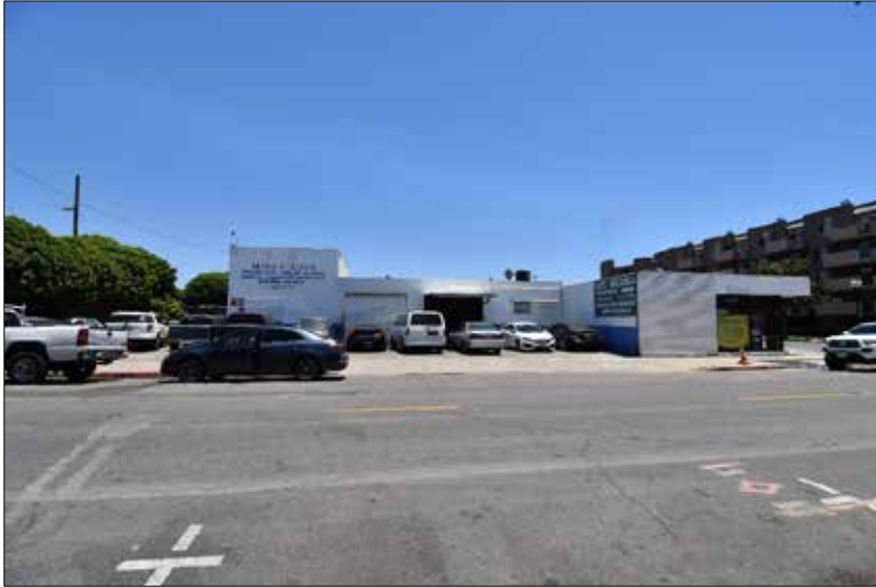
Southwest View of Site B from 4th Street and Mortimer Street
