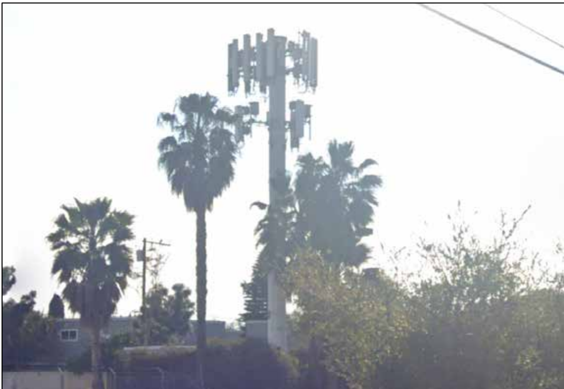
2120 South Bristol Street – Co-location
