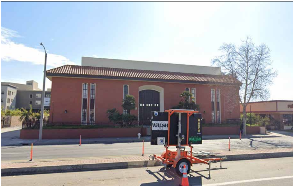
3636 Westminster Avenue – Roof mounted antennas
