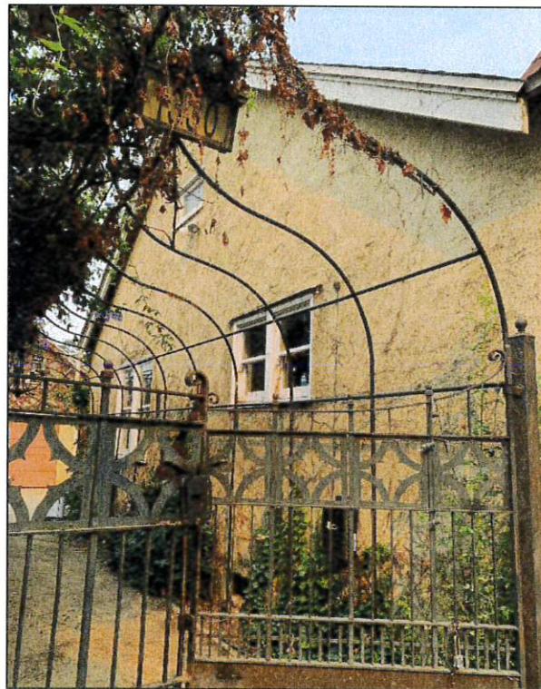
HPPA-2020-01 WAHL HOUSE 1330 SOUTH BROADWAY SITE PHOTOS EXHIBIT 3
