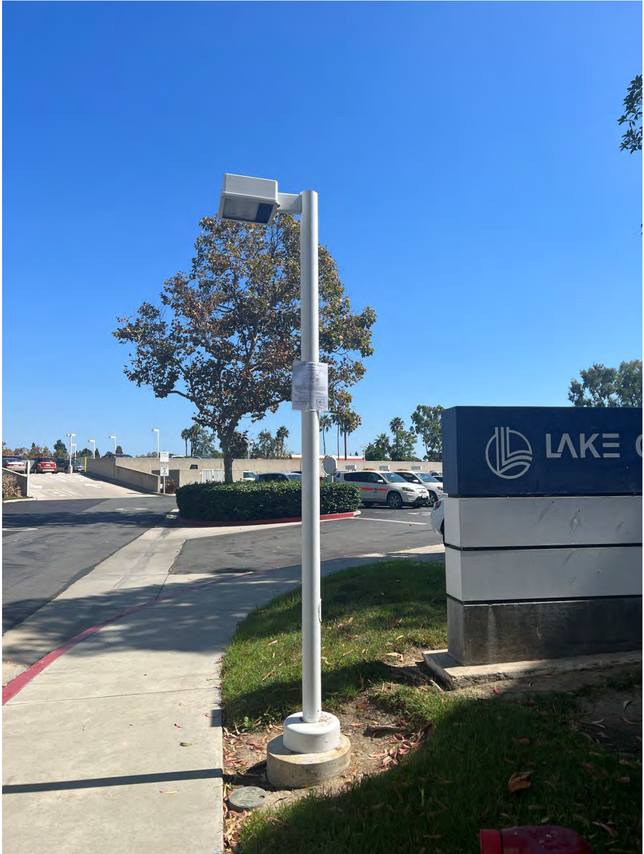
W. Lake Center Drive – eastern entry driveway
