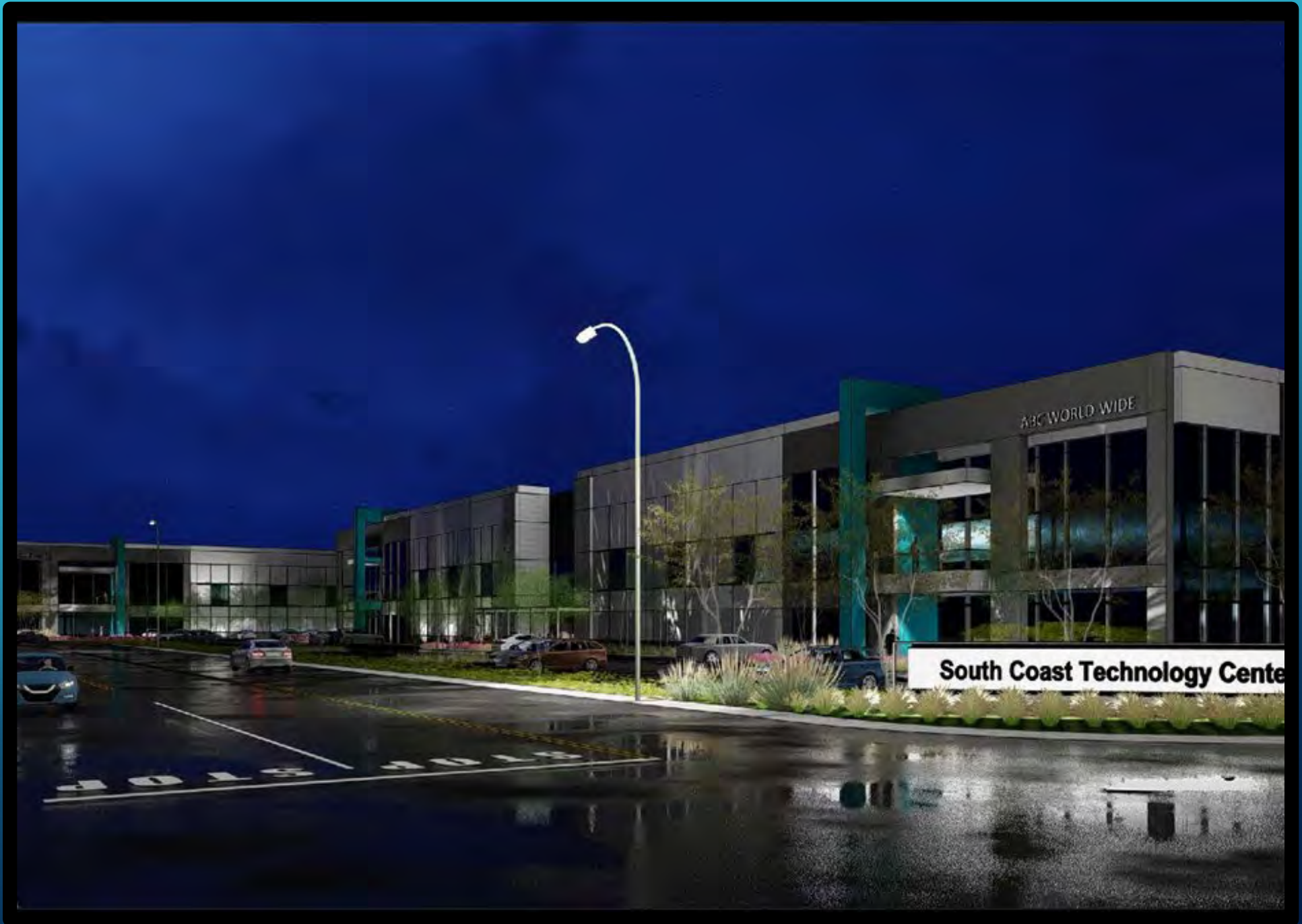
SOUTH COAST TECHNOLOGY CENTER
