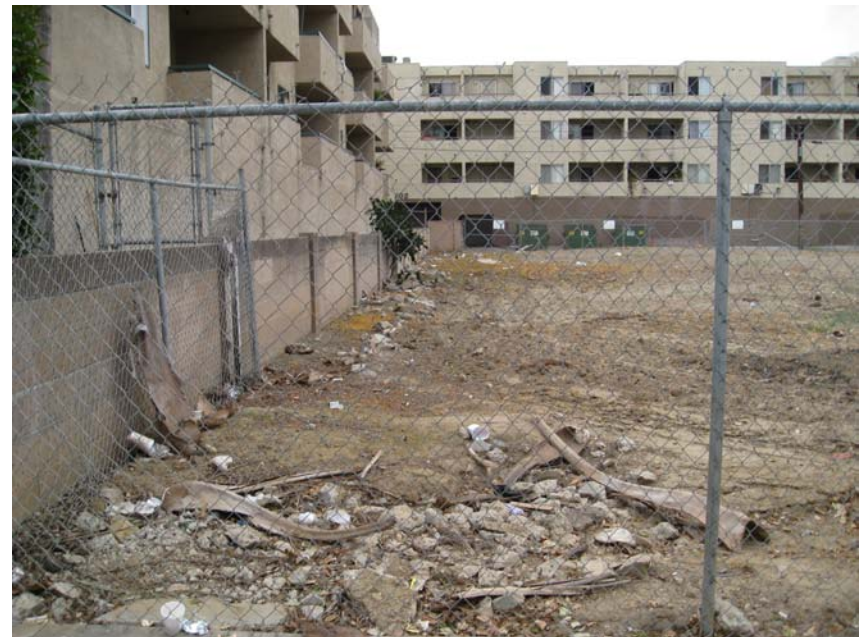
View of the debris observed at the southeast corner of the Property.
