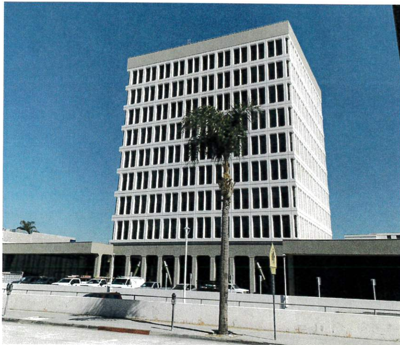
HPPA-2020-17 SECURITY BANK BUILDING 888 NORTH MAIN STREET SITE PHOTOS EXHIBIT 3
