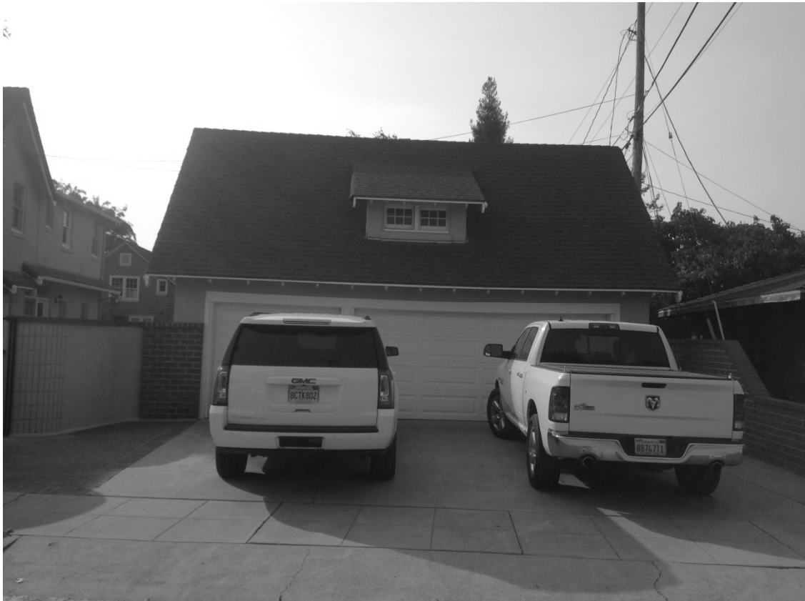
#5 East Elevation – Benton Way
