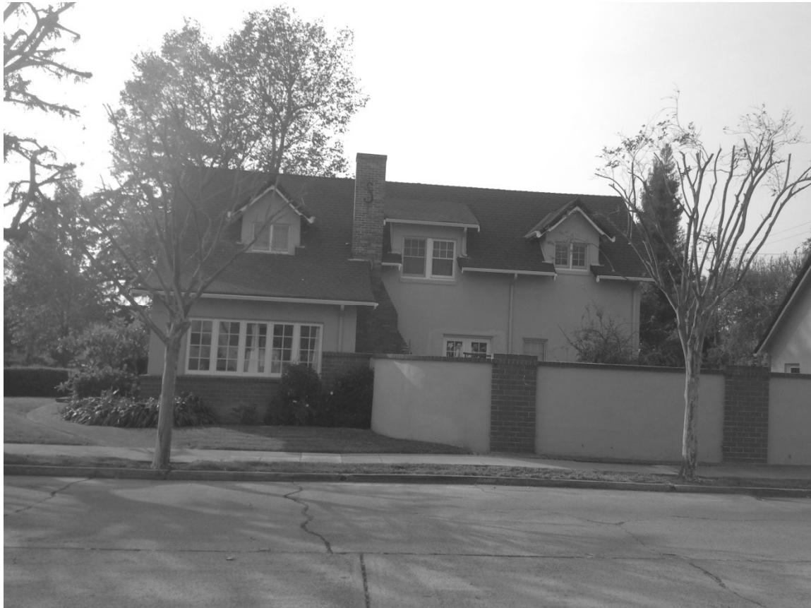
#2 East Elevation – Benton Way
